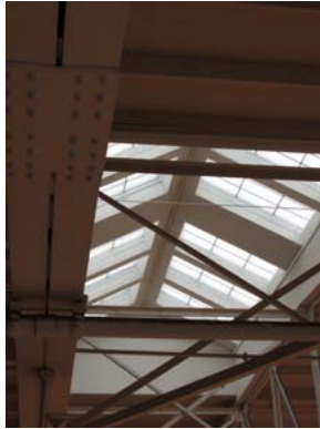
Between the skylights and tall windows, the old gym has lots of natural light.
